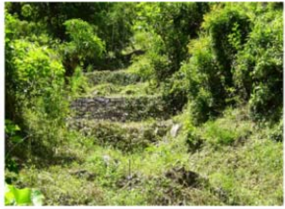
Sausage wall with Bio-engineering measures protected the agricultural land
