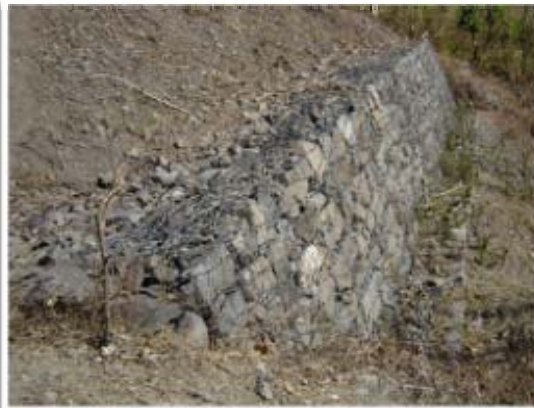
Series of sausage wall built to retain the soil
