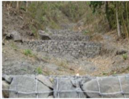
Series of sausage wall built to retain the soil
