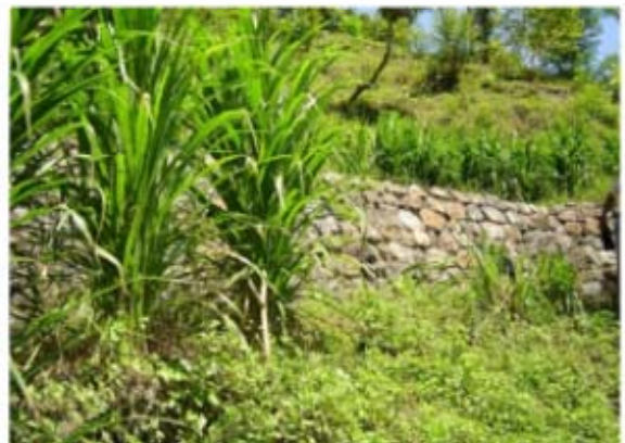
Sausage wall with Bio-engineering measures protected the agricultural land
