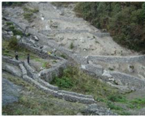
During Treatment: Hand packed stone wall inside sausage being built
