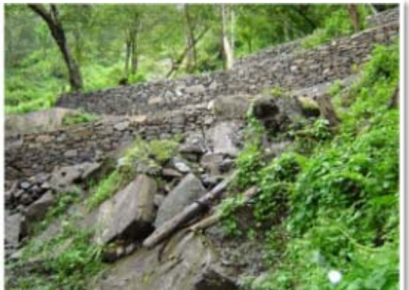
Landslide Site brought under control with gabion structures
